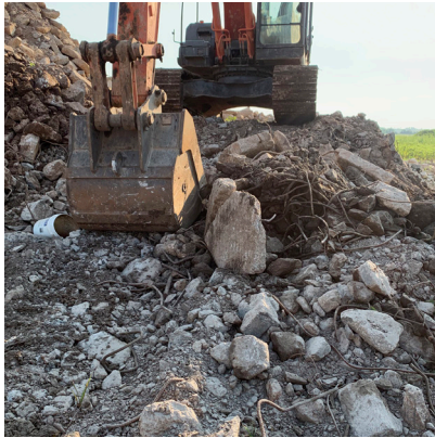
ROAD BASE WITH REBAR
